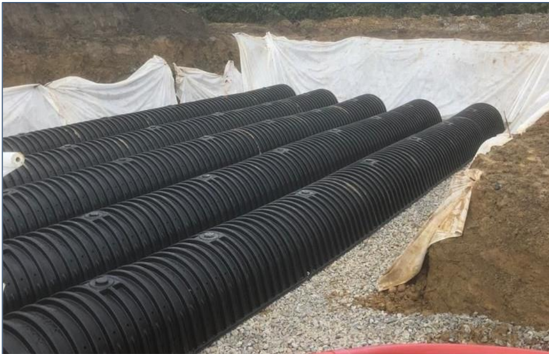
Figure 4-9 Typical Poly Tunnel Installation Arrangement
